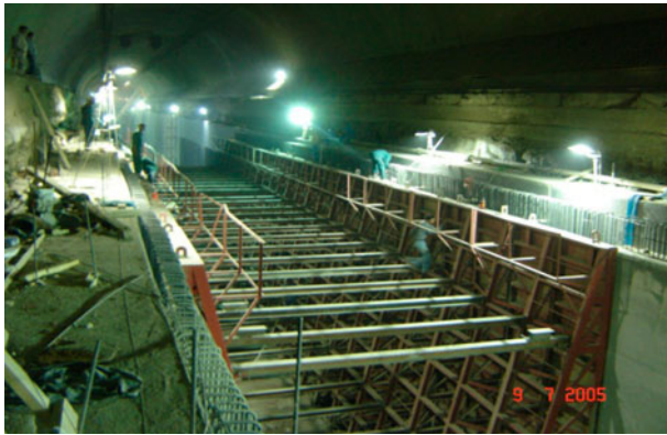
Fig. 2. Side forms of tunnel segment
