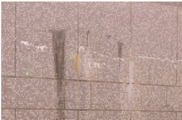
Figure 6. The close-range horizontal photography by UAV's camera
