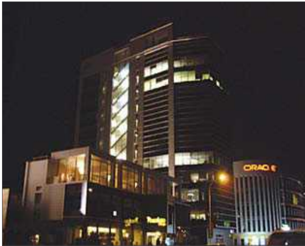
16 pav. Administraciniai pastatai naktį Goštauto g. Fig. 16. Administration buildings at night in Goštautas str
