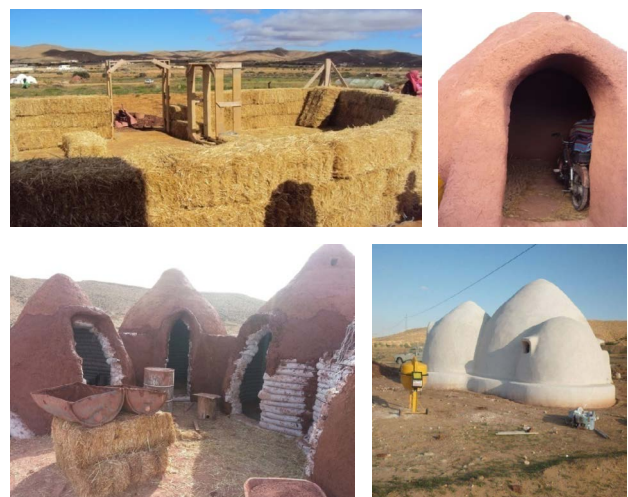
Figure 7. The eco-dom: Local attempts at design with vernacular bioclimatic references, Oued El Khil, Governorate of Tataouine (Toumi, 2018)
