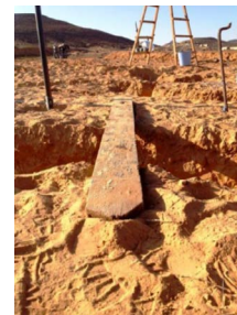
Figure 15. Leveling the trench with a drywall's spirit level (Toumi, 2019c)
