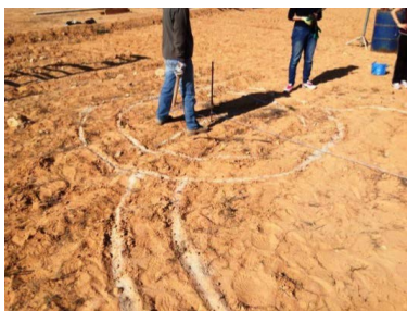
Figure 13. Tracing the dome on the ground (Toumi, 2019c)
