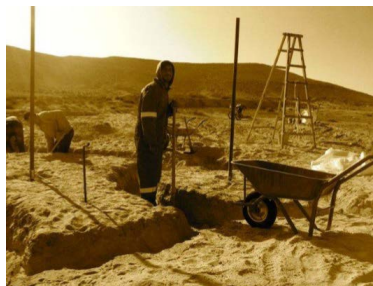
Figure 14. Digging of trenches (Toumi, 2019c)
