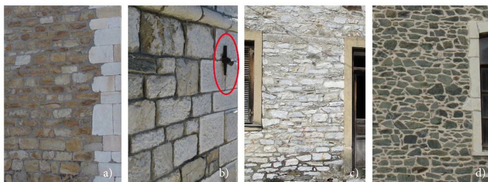
Figure 11. Masonry types of the stone schools: a) Arnaia, 1871; b) Stratoniki, 1904; c) Varvara, 1909; d) M. Panagia, 1932 (source: author)
