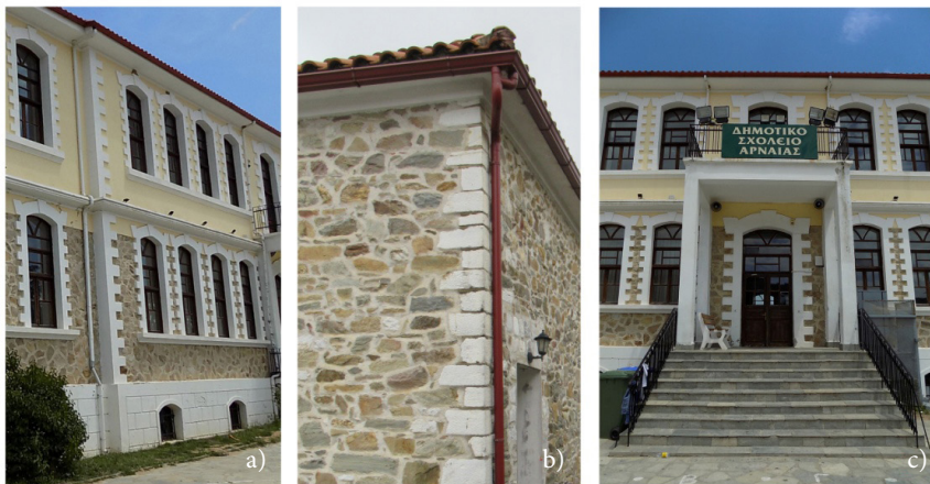
Figure 9. Other architectural aspects: a) Perimetric horizontal stripes in Arnaia, 1931; b) Ashlar cornerstones in Neochori, 1947; c) Central entrance shelter in Arnaia, 1931 (source: author)
