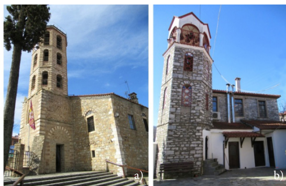
Figure 5. Attachment of the church's tower bell on the back side of the schools (pictures taken from the churches' courtyard): a) Arnaia, 1871; b) Varvara, 1909 (source: author)
