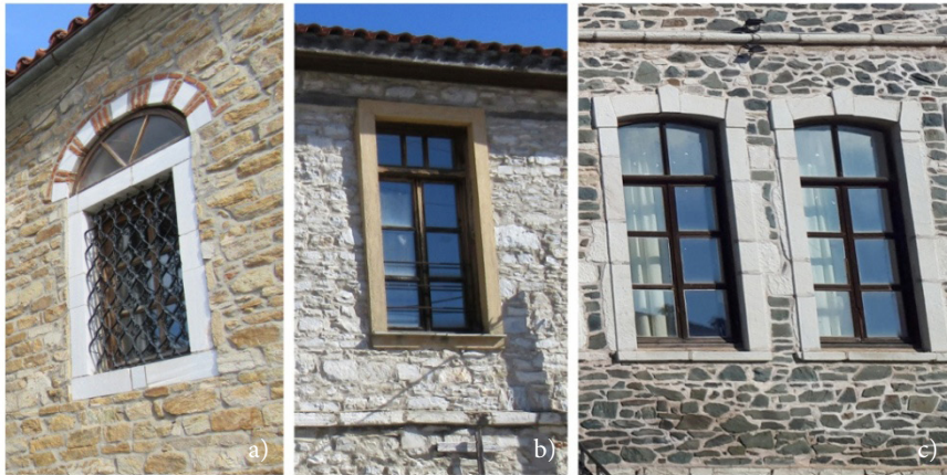
Figure 8. Openings' types of the stone schools: a) Arnaia, 1871; b) Varvara, 1909; c) M. Panagia, 1932 (source: author)
