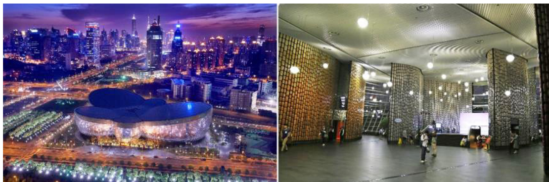
Figure 8. Oriental Art Center, building and lobby
