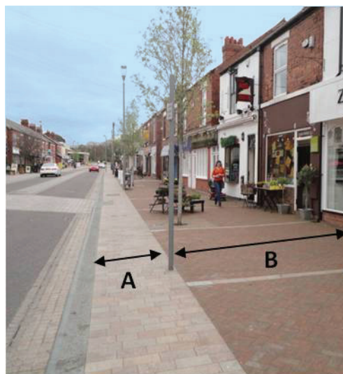
Figure 6. Pedestrian safe area in Park Lane
