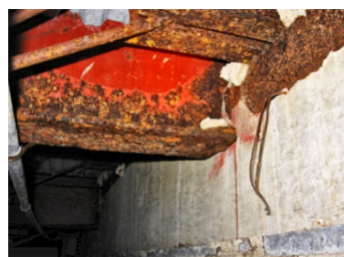
Fig. 9. Damaged beams
