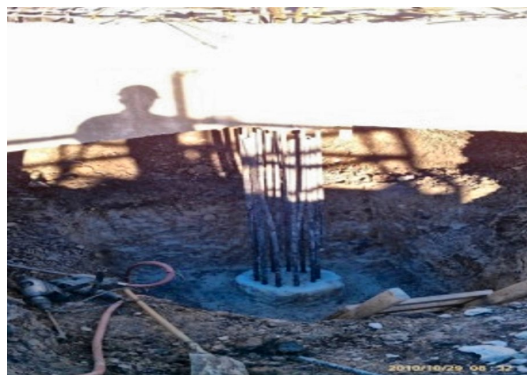
Fig. 12. Grade beam over exposed pier
