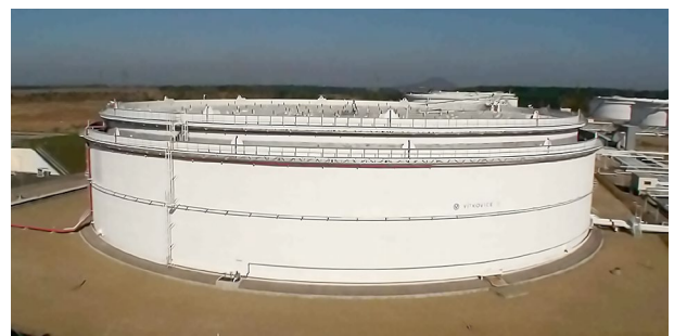
Fig. 1. Welded tank for oil storage
