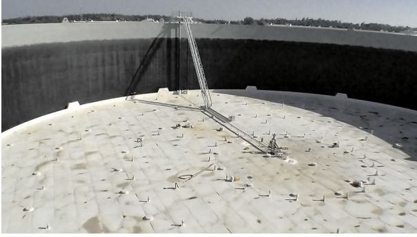
Fig. 2. Floating roof in a drained tank
